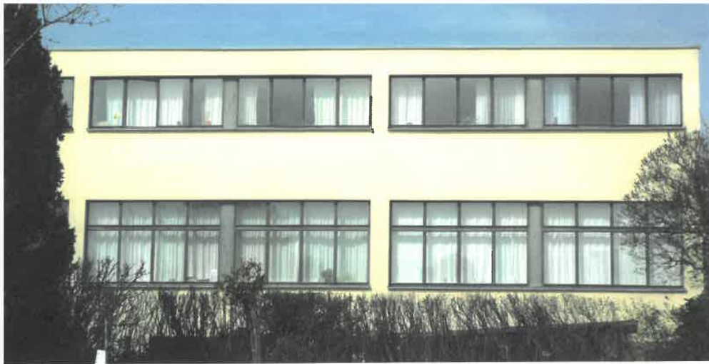
Häuser Stam, Gartenansicht, 2016 / Stam Houses, garden view, 2016
